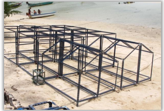
Picture 1: Coral Nursery tables after construction
